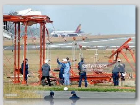
approach to runway 28 on 14 April. It hit an approach light at a height of 4m before carving through the antenna. Flight OZ162 subsequently veered off the runway, suffering substantial airframe damage.
